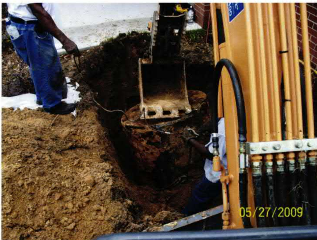
Picture 2: UST 1041Gardenia during removal.
